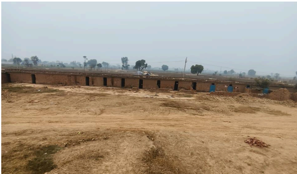
3-meter high boundary wall
